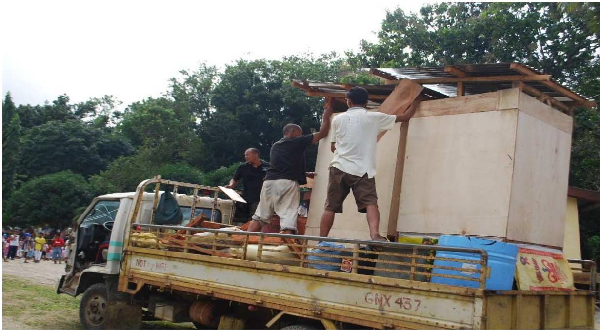
Transporting portable ecosan toilets and installing it where the victims are located.
